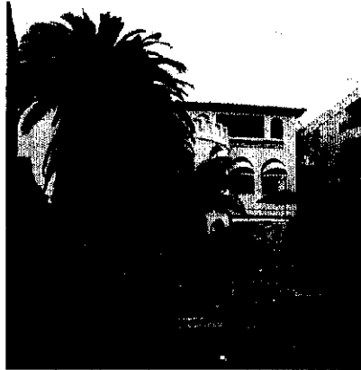
Figure 11: 2005 view of the north elevation showing the 1972 alterations, including the second floor addition to original bow front (left), and the 1972 single-storey bow front (right).
