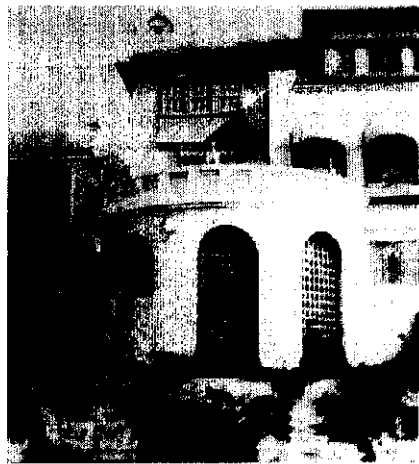
Figure 9: Detail of the single-storey Moderne style bow front featuring lattice covered arched openings, early 1930s. This space is now part of two flats. (Source: Manly Warringah and Pittwater Historical Society)
